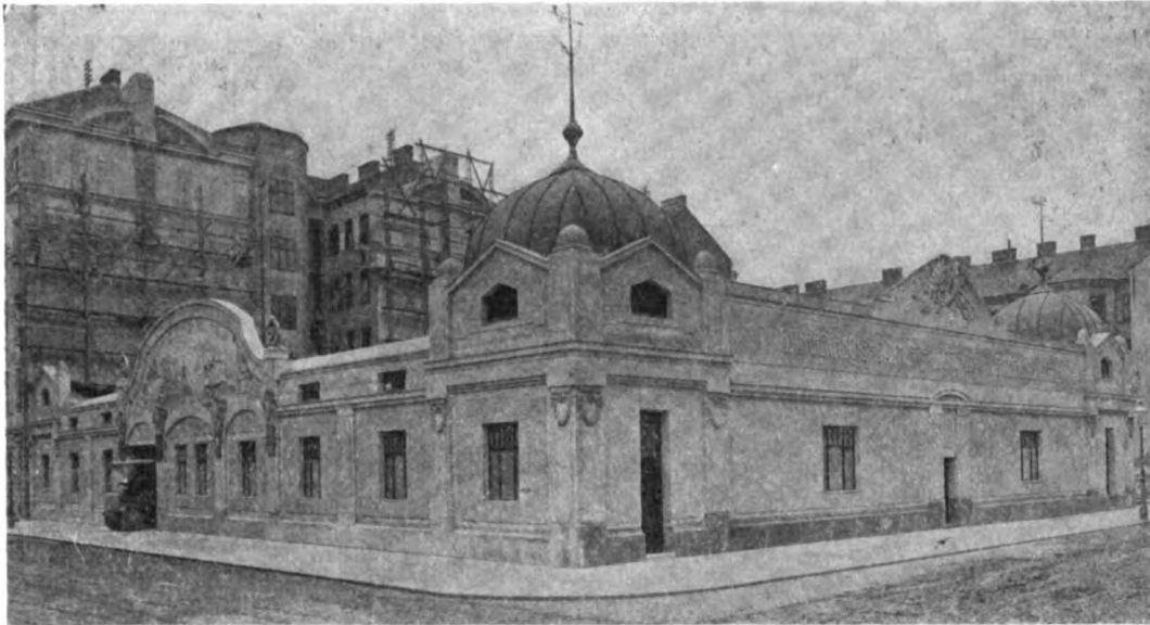
Where the electric mail vans are garaged in Vienna. The building is 131 by 102 feet, of one story and basement, and fronts on three streets. The interior, together with the idea of stalls for the cars, is illustrated below
